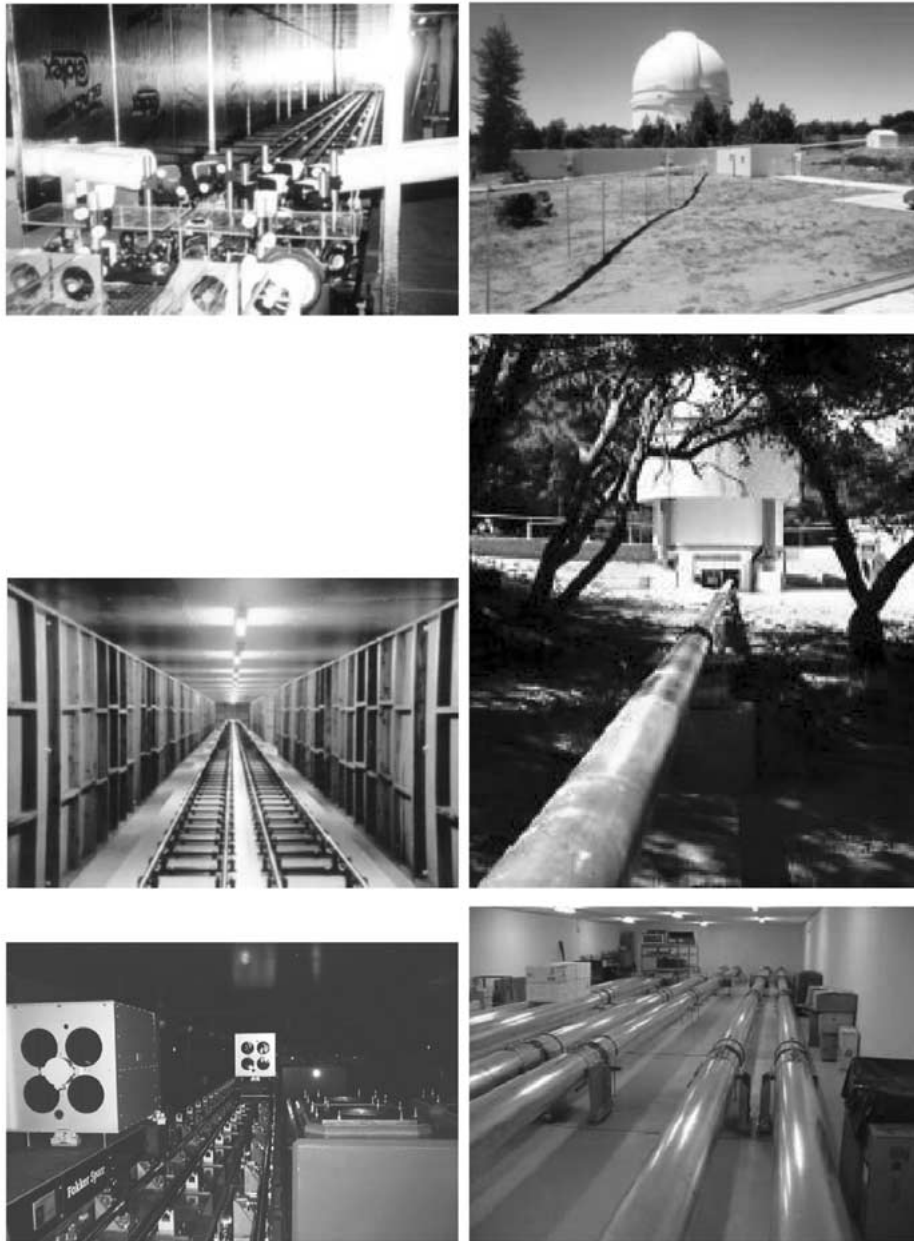
Figure 6. Beam transport in interferometers can run through open air or within evacuated pipes. The left column shows the air tunnels of PTI, SUSI and VLTI (the first two building-in-building, the latter a wine cellar). The right column shows the pipes of PTI and the pipes of CHARA outside and inside the interferometric building (both from top to bottom).
